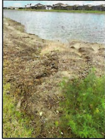
Picture 2: Large erosion trails >20' wide
