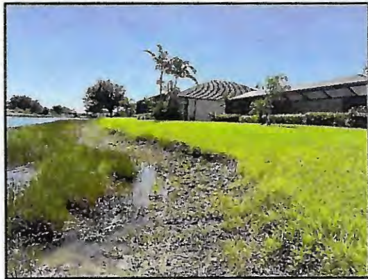
Picture 3: >8" T.O.B erosion
