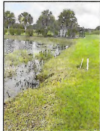
Picture 3: >8" T.O.B erosion (~160 LF)
