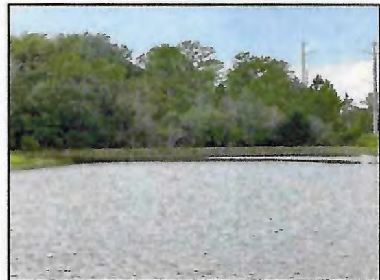
Picture 5: >8" T.O.B erosion (~230 LF)
