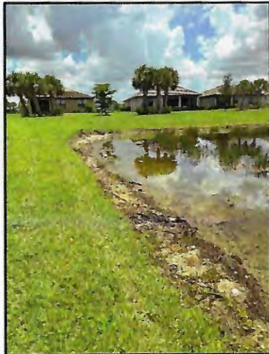
Picture 3: 6-8" T.O.B erosion (~418 LF)
