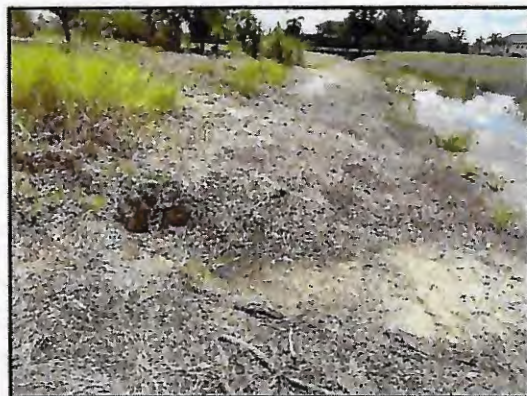
Picture 3: Large washout within bank
