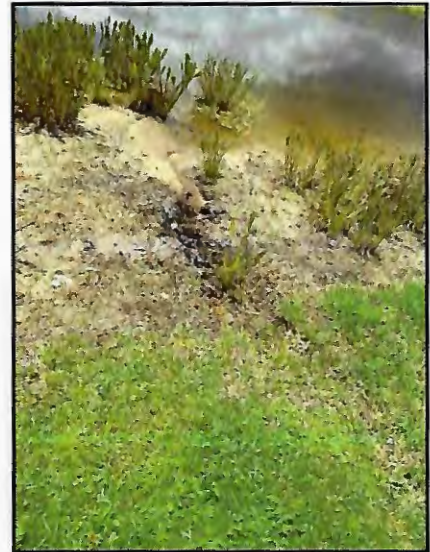
Picture 4: Washout from roof leader
