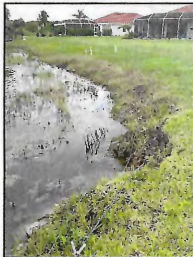
Picture 2: >8" T.O.B erosion (~100 LF)
