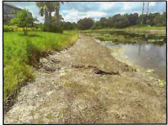
Picture 4: Large washout with TOB erosion
