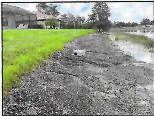
Picture 1: Disconnected PVC yard drain
