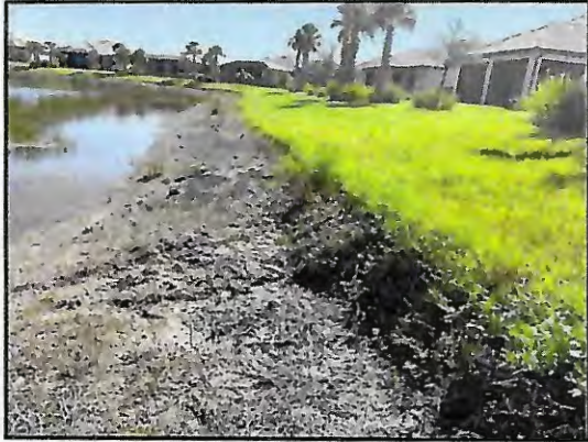
Picture 5: >8" T.O.B erosion
