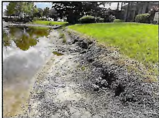
Picture 3: >8" T.O.B erosion with washout
