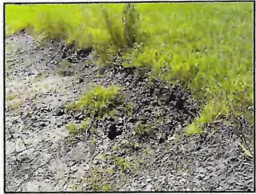
Picture 2: >8" T.O.B erosion
