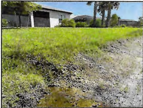
Picture 3: >8" T.O.B erosion ; steep bank slope
