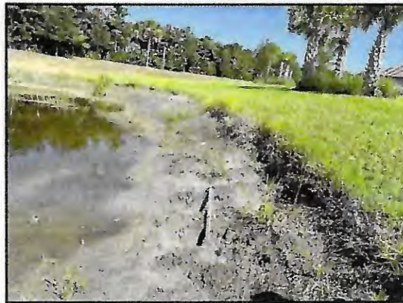
Picture 7: >8" T.O.B erosion
