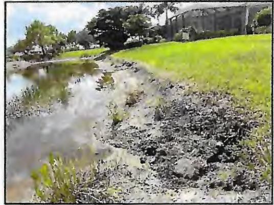
Picture 2: >8" T.O.B erosion with washout
