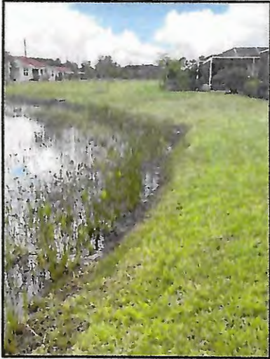
Picture 1: >8" T.O.B erosion (~72 LF)
