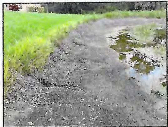
Picture 2: >8" T.O.B erosion
