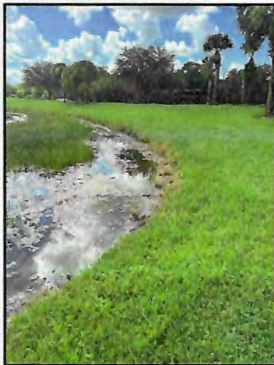
Picture 3: >8" T.O.B erosion
