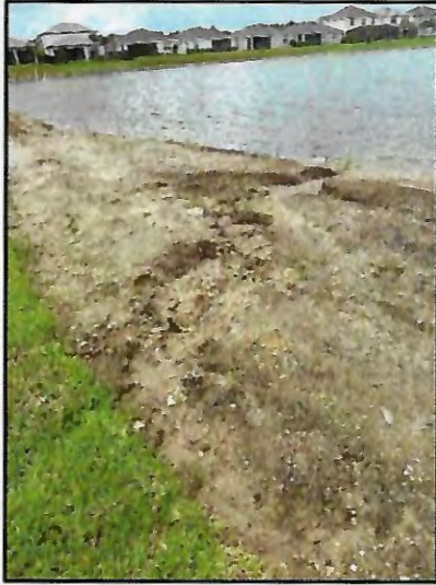
Picture 1: Large erosion trails >20' wide
