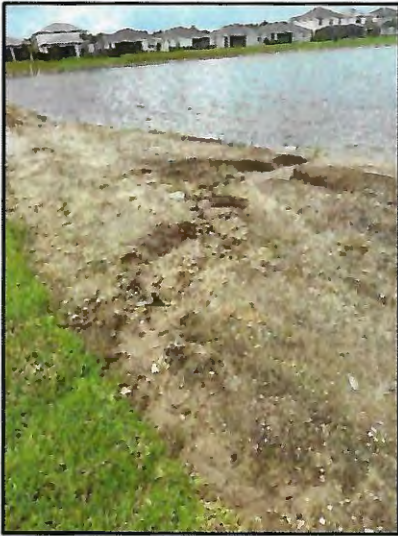
Picture 1: Large erosion trails >20' wide
