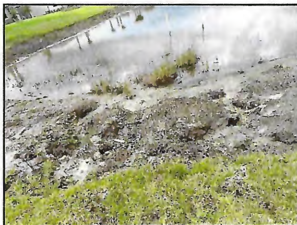
Picture 3: Large length of washout
