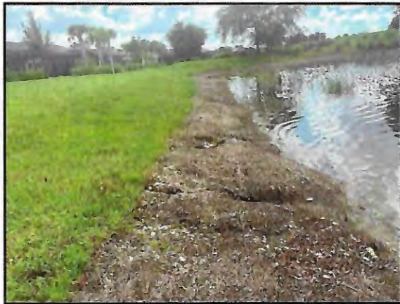
Picture 3: Forming washout trails
