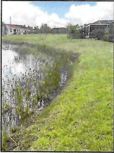
Picture 1: >8" T.O.B erosion (~72 LF)
