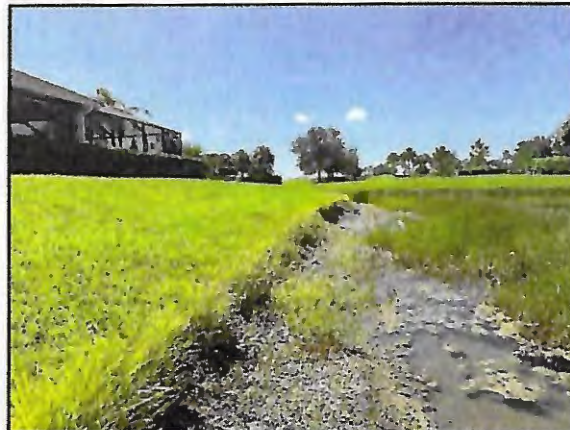
Picture 2: >8" T.O.B erosion
