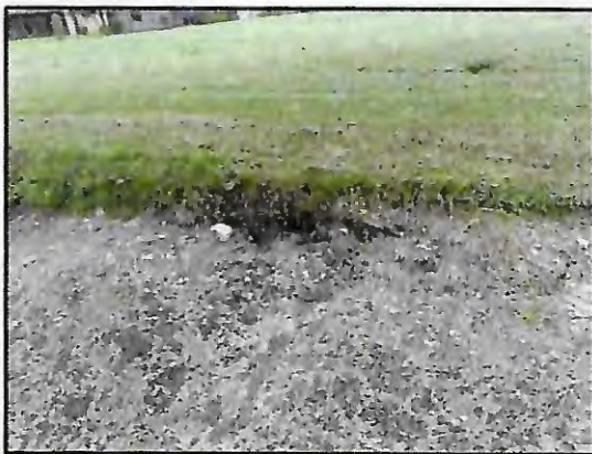
Picture 5: Washout forming under bank
