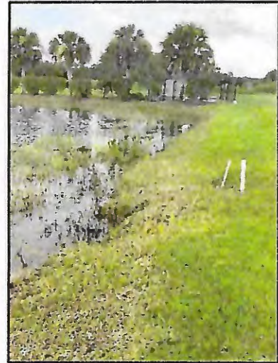
Picture 3: >8" T.O.B erosion (~160 LF)
