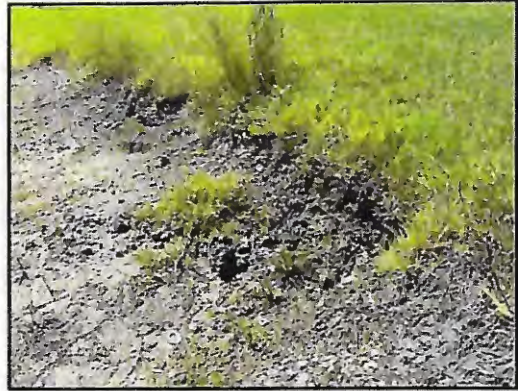
Picture 2: >8" T.O.B erosion
