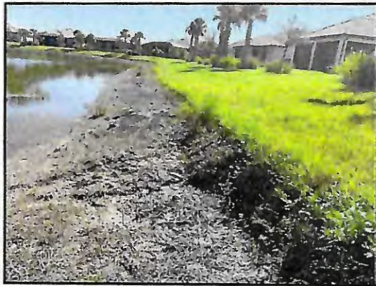
Picture 5: >8" T.O.B erosion (~166 LF)
