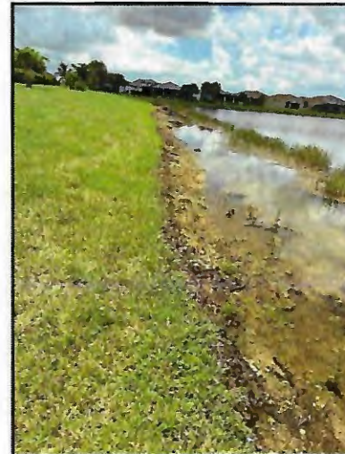
Picture 4: >8" T.O.B erosion (~600 LF)
