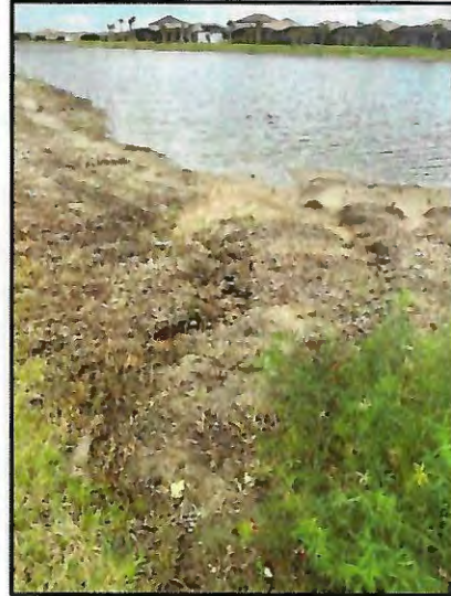
Picture 2: Large erosion trails >20' wide
