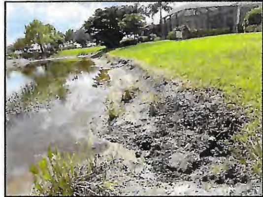
Picture 2: >8" T.O.B erosion with washout
