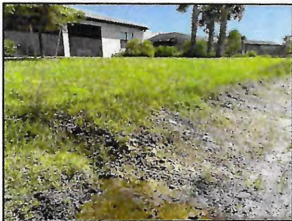
Picture 3: >8" T.O.B erosion ; steep bank slope
