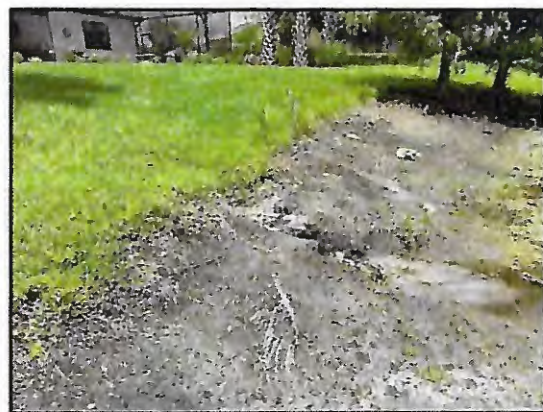
Picture 6: Large washout from irrigation
