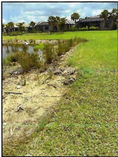
Picture 3: 6-8" T.O.B erosion (~260 LF)
