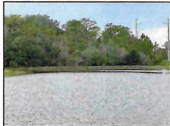
Picture 5: >8" T.O.B erosion (~230 LF)
