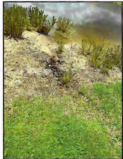
Picture 4: Washout from roof leader
