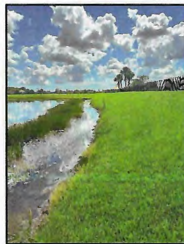
Picture 4: >8" T.O.B erosion (~420 LF)
