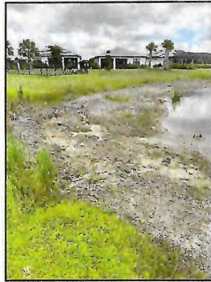
Picture 5: 6-8" T.O.B erosion
