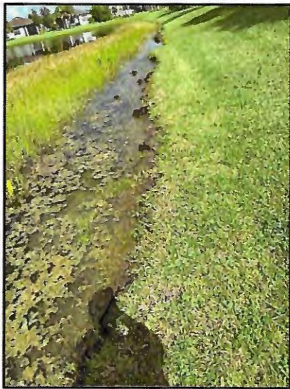
Picture 1: 6-8" T.O.B erosion
