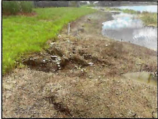
Picture 1: Large washout with TOB erosion
