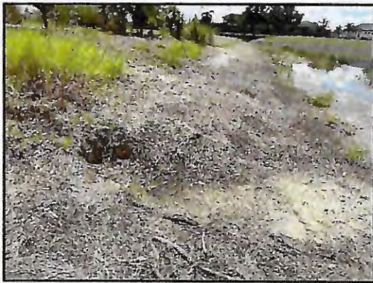
Picture 3: Large washout within bank
