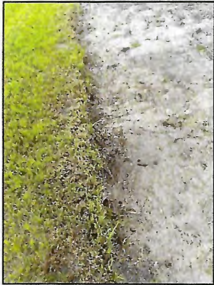
Picture 1: >8" T.O.B erosion
