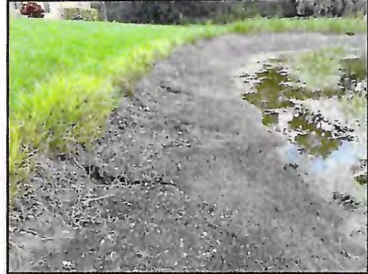
Picture 2: >8" T.O.B erosion
