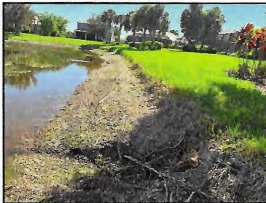
Picture 2: >8" T.O.B erosion (~193 LF)
