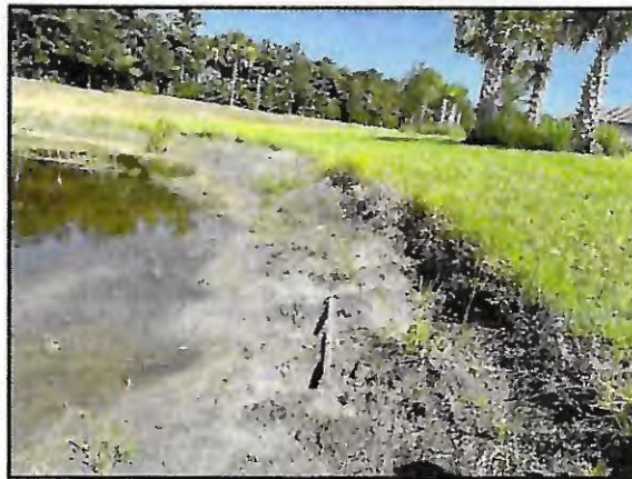
Picture 7: >8" T.O.B erosion (~388 LF)
