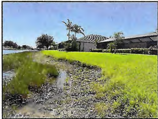
Picture 3: >8" T.O.B erosion
