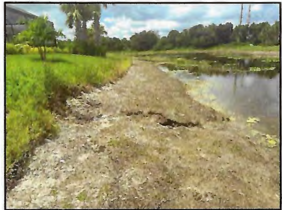
Picture 4: Large washout with TOB erosion
