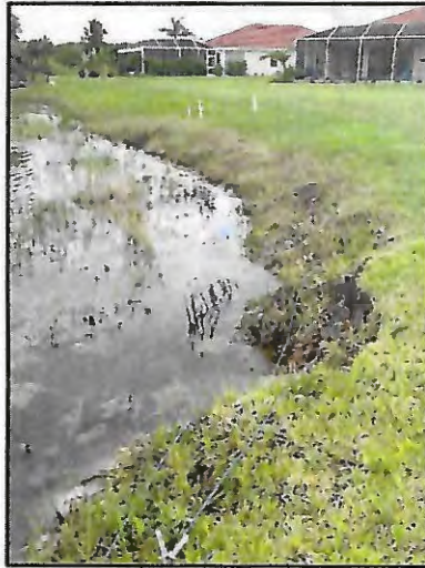
Picture 2: >8" T.O.B erosion (~100 LF)
