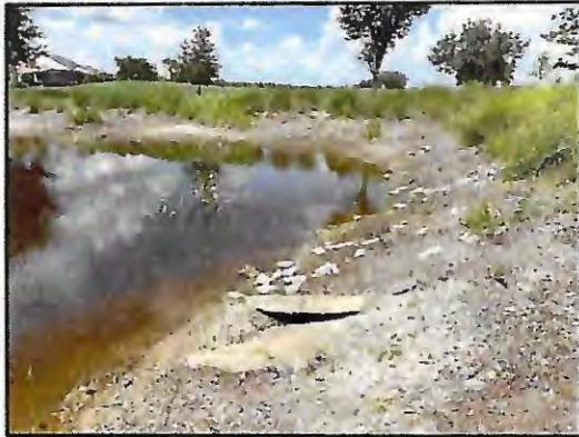
Picture 1: >8" T.O.B erosion
