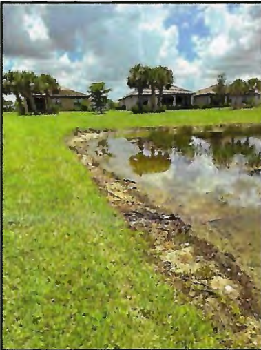
Picture 3: 6-8" T.O.B erosion (~418 LF)
