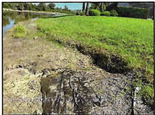
Picture 3: Large washout washout
