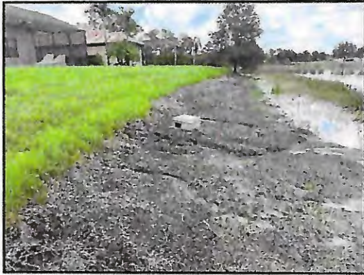
Picture 1: Disconnected PVC yard drain
