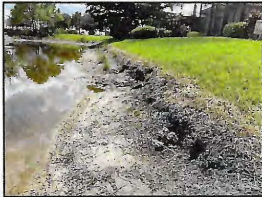
Picture 3: >8" T.O.B erosion with washout
