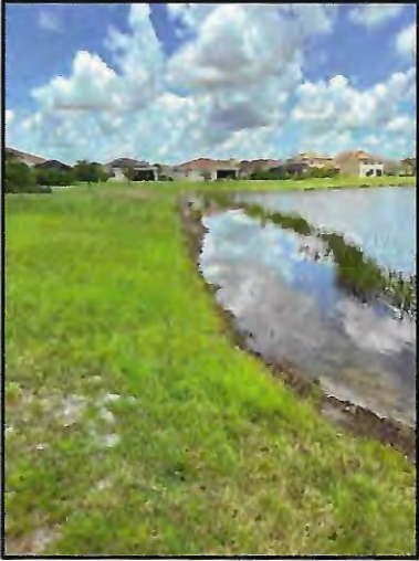
Picture 1: >8" T.O.B erosion (~160 LF)
