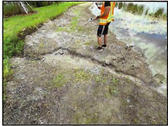
Picture 2: Large washout with TOB erosion
