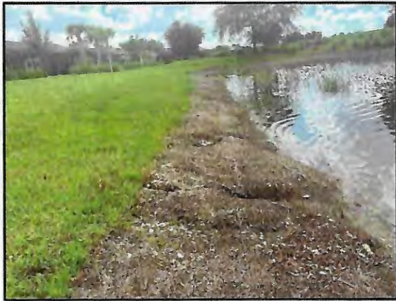
Picture 3: Forming washout trails
