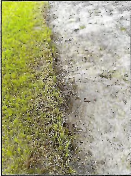
Picture 1: >8" T.O.B erosion
