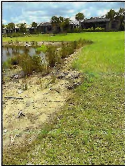
Picture 3: 6-8" T.O.B erosion
