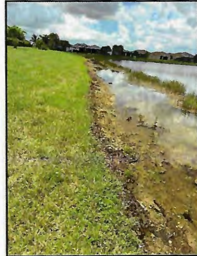
Picture 4: >8" T.O.B erosion (~600 LF)
