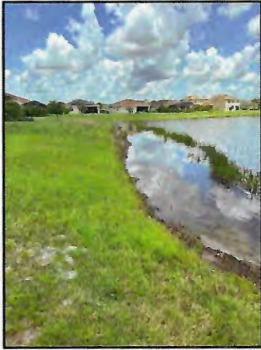
Picture 1: >8" T.O.B erosion (~160 LF)
