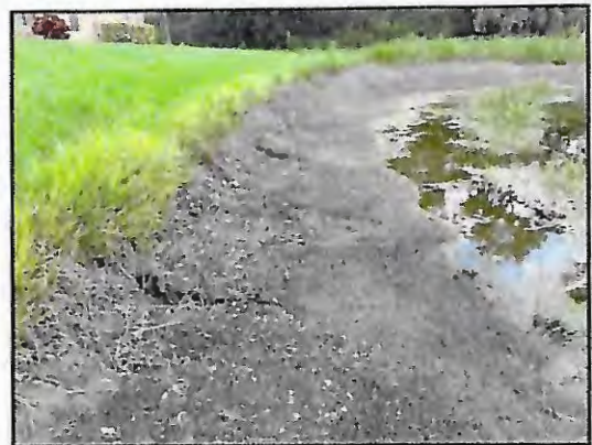
Picture 2: >8" T.O.B erosion
