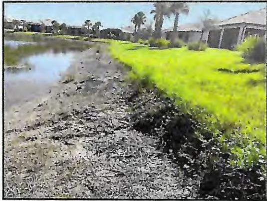
Picture 5: >8" T.O.B erosion
