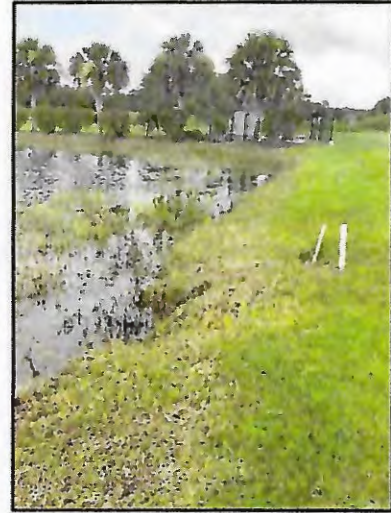
Picture 3: >8" T.O.B erosion (~160 LF)
