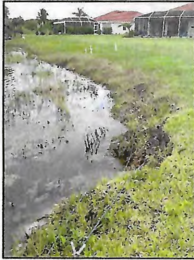
Picture 2: >8" T.O.B erosion (~100 LF)
