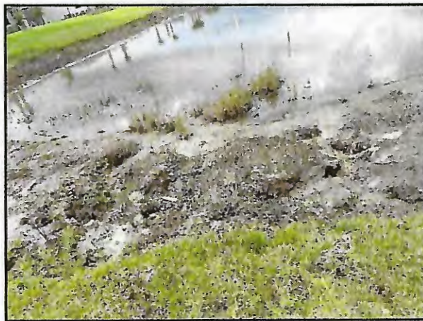
Picture 3: Large length of washout
