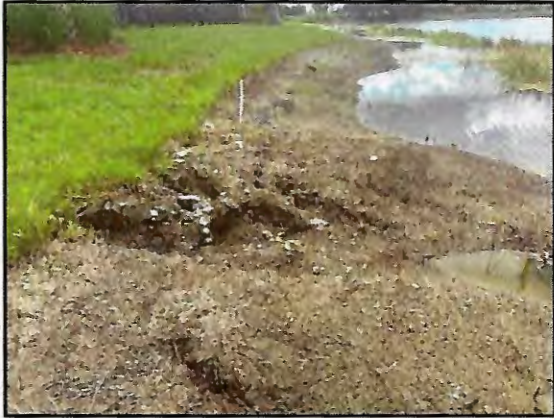
Picture 1: Large washout with TOB erosion
