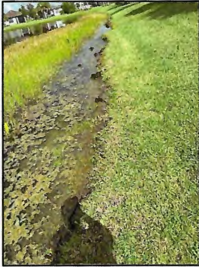
Picture 1: 6-8" T.O.B erosion
