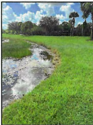
Picture 3: >8" T.O.B erosion
