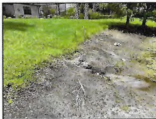
Picture 6: Large washout from irrigation
