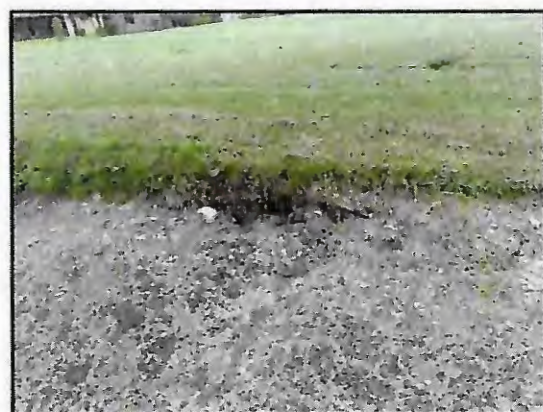
Picture 5: Washout forming under bank
