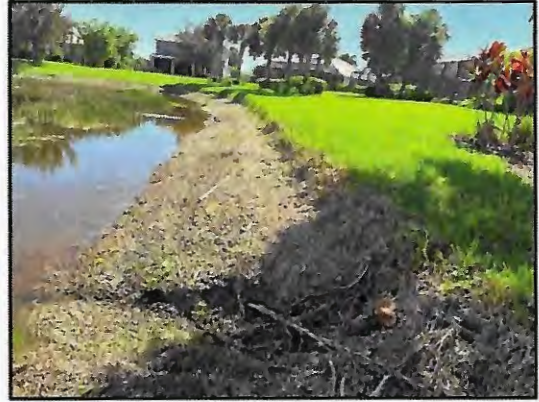
Picture 2: >8" T.O.B erosion
