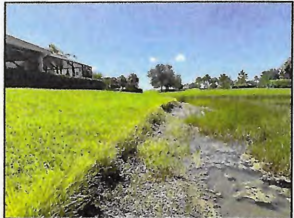
Picture 2: >8" T.O.B erosion
