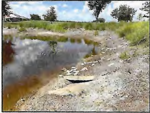
Picture 1: >8" T.O.B erosion
