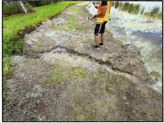
Picture 2: Large washout with TOB erosion
