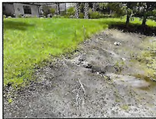
Picture 6: Large washout from irrigation
