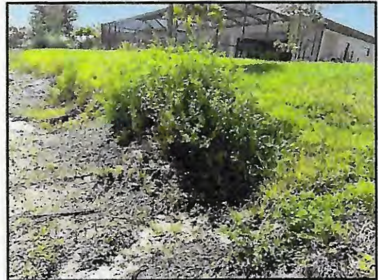
Picture 4: >8" T.O.B erosion
