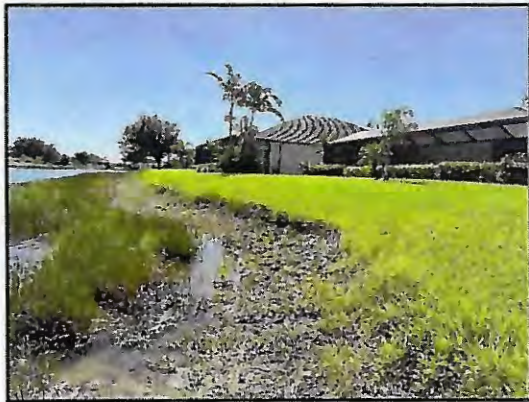
Picture 3: >8" T.O.B erosion
