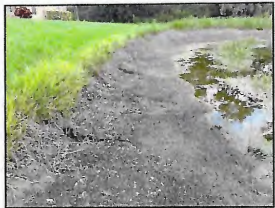
Picture 2: >8" T.O.B erosion
