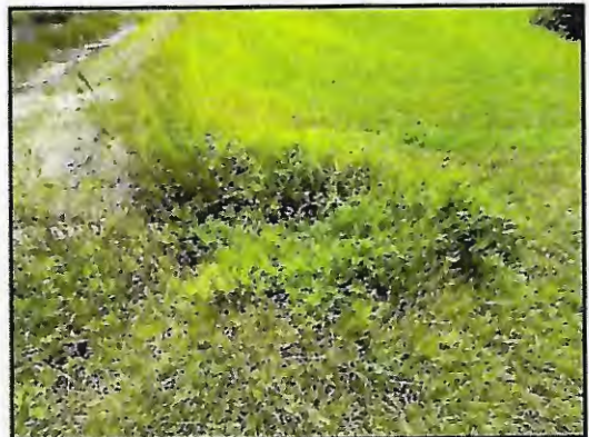
Picture 6: >1' deep washout
